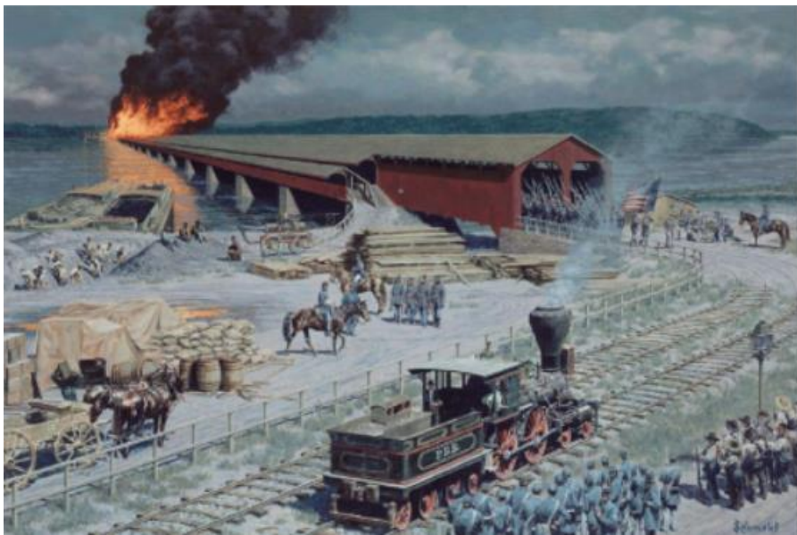
The burning of the Wrightsville bridge. Painting by Bradley Schmehl.
